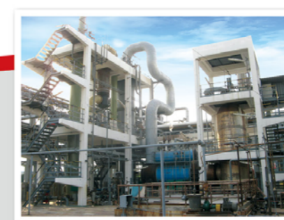
氯碱装置焚烧单元 (上海氯碱三期) Incineration unit of waste gas and liquid containing chlorofluorocarbon (phase III of Shanghai Chloro-alkali Plant)
