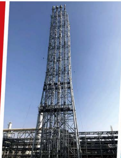
可拆卸式高架火炬 (高度 100m, 浙石化) Demountable elevated flare (H=100m, Zhejiang Petrochemical)
