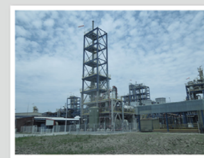
氟化工废气废液焚烧单元 (阿科玛) Incineration unit of waste gas and liquid containing fluorine (ARKEMA)
