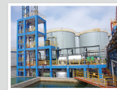
氟化工废气废液焚烧单元 (江苏三爱富) Incineration unit of waste gas and liquid containing fluorine (Changshu 3F)
