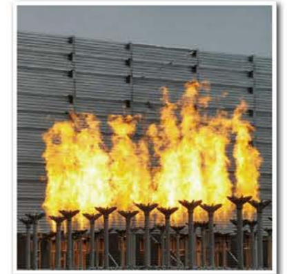
开放式地面火炬燃烧运行 Multi-burner staged flare combustion operation
