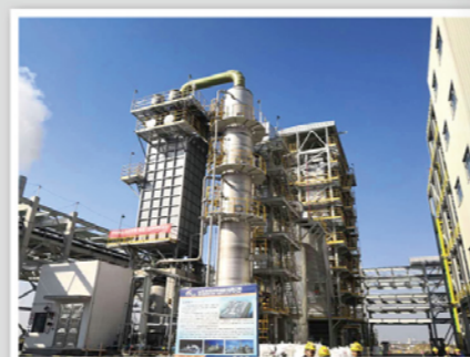
氨基酸钾盐废液焚烧装置 (山东新和成) Incineration unit of Potassium amino acid salt waste liquid (Shandong Xinhecheng)
