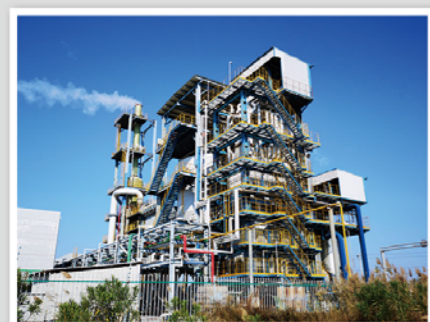
农药废气废液焚烧单元 (南通雅本) Incineration unit of waste gas and liquid in pesticide industry (Nantong Yaben)
