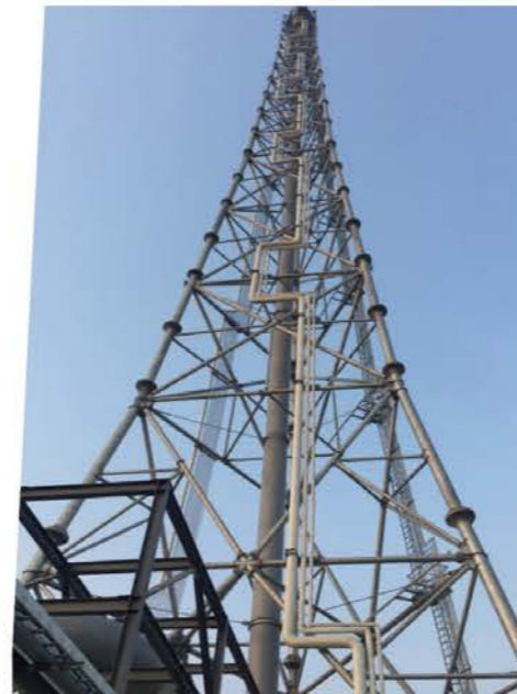
捆绑式高架火炬 (高度 150m, 河北海伟) Multi-stack elevated flare (H=150m, Hebei Haiwei)
