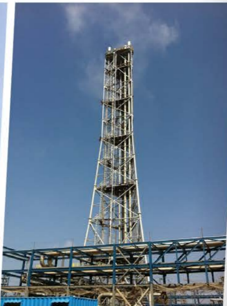
捆绑式高架火炬 (高度 100m, 江苏尔邦) Multi-stack elevated flare (H=100m, Jiangsu Sierbang)
