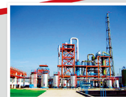
有机硅废气废液焚烧单元 (山东东岳二期) Incineration unit of waste gas and liquid containing chlorosilane (Phase II of Shandong Dongyue)
